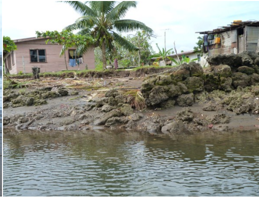
At low tide, Headman, Sailosi Ramatu points out the effects of coastal erosion and where the seawall has been breached. The seawall used to protect Vunidogoloa.
